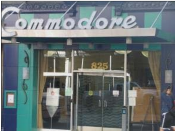
Photograph 79. Main entryway to ES-14.
