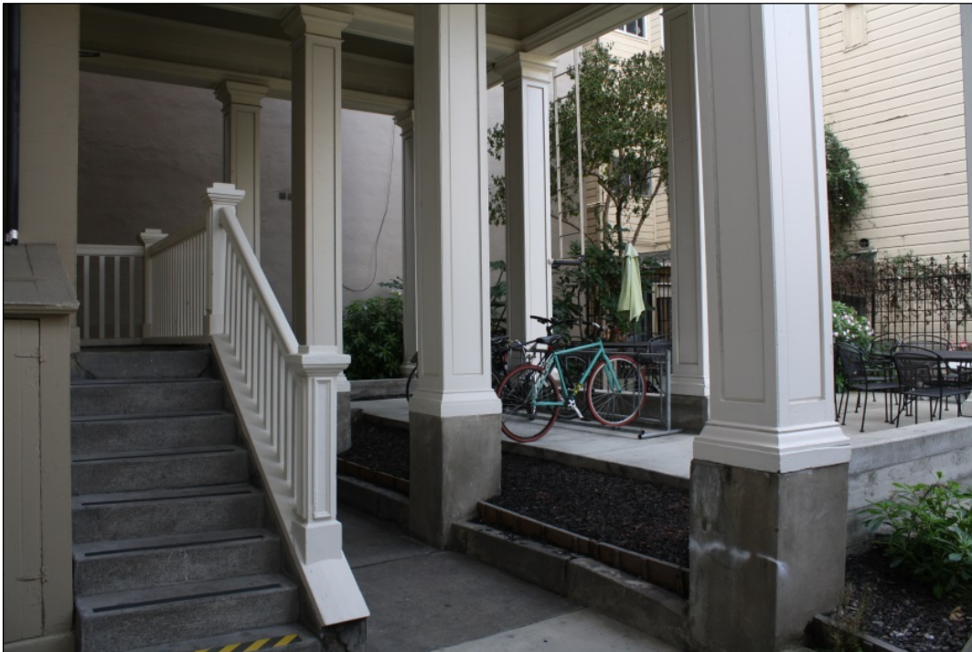
Figure 339. 2209 Van Ness Avenue, view of the columns under the second story addition and the rear patio.
