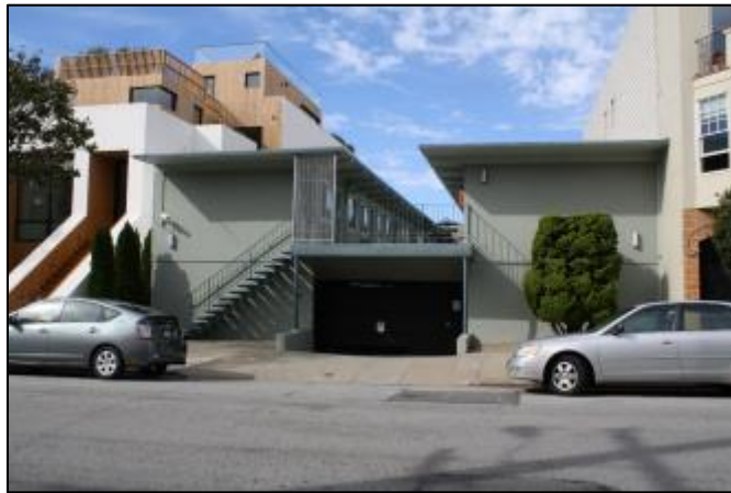
Photograph 20. Rear (south) façade, Star Motel, 1727 Lombard Street
