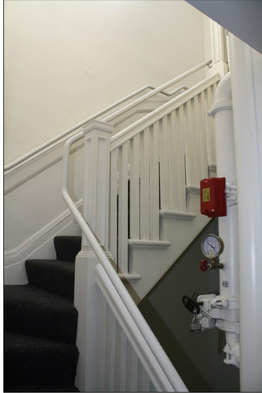
Figure 178. Interior stair of subject property.
