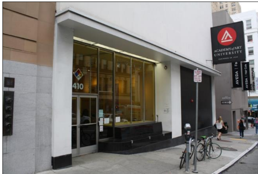
Figure 2. 410 Bush Street, detail, first story of the primary elevation. (Source: SWCA)
