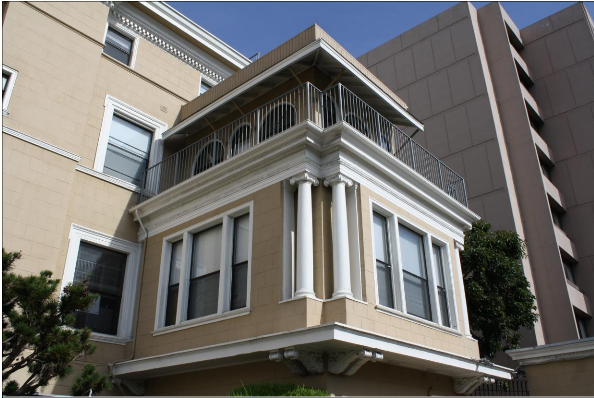
Figure 8. Three-story addition at south façade, 1916 Octavia Street. Source: SWCA, 2015.
