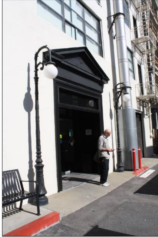
Figure 49. 58-60 Federal Street, detail, main entrance, primary elevation (Source: SWCA)
