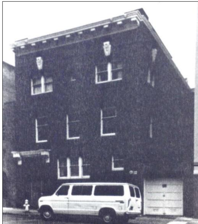
Figure 38. 1978 photo 1153 Bush Street. (Source: San Francisco Architectural Heritage Survey)
