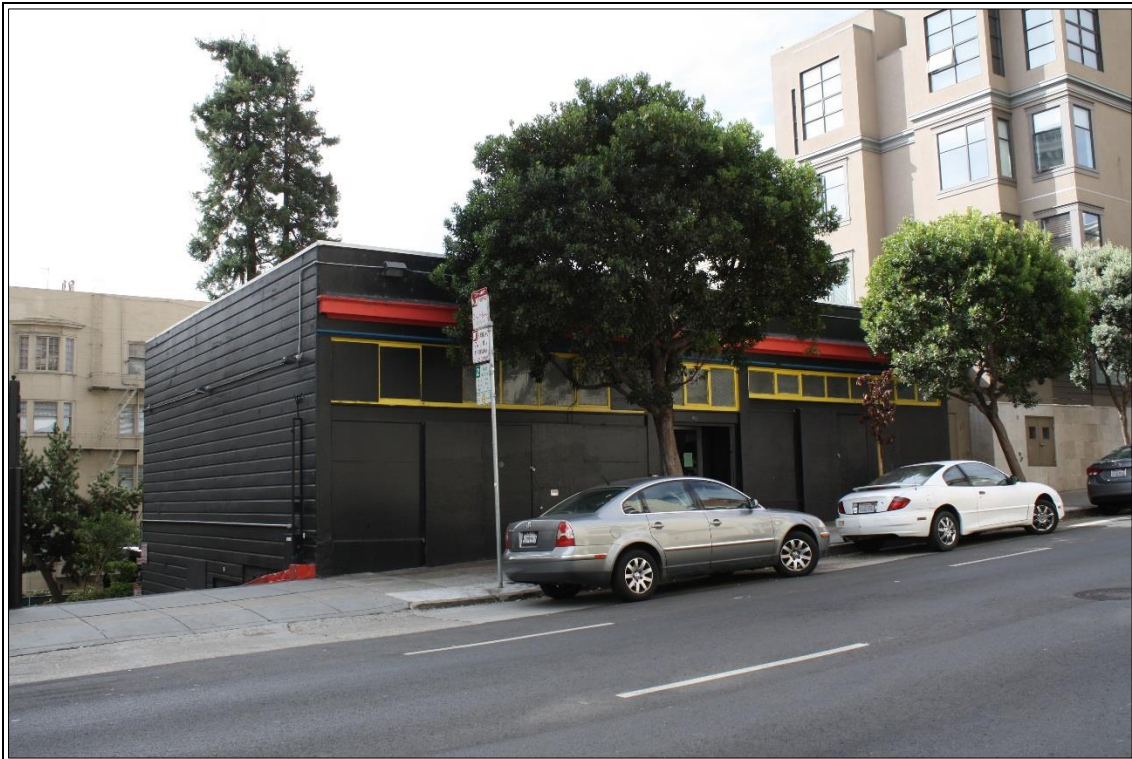
Figure 4. North façade, 1069 Pine Street. Source: SWCA, 2015.
