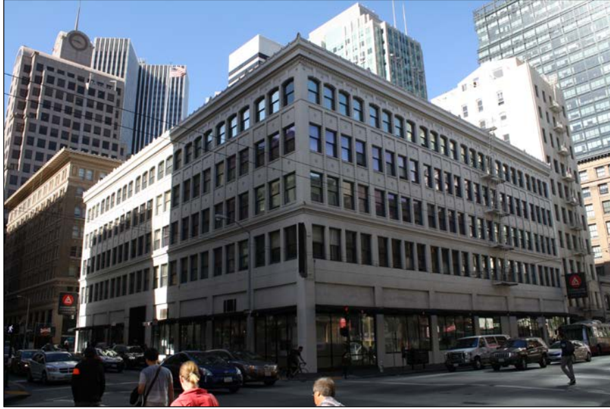
Figure 58. 77-79 New Montgomery Street. (Source: SWCA)
