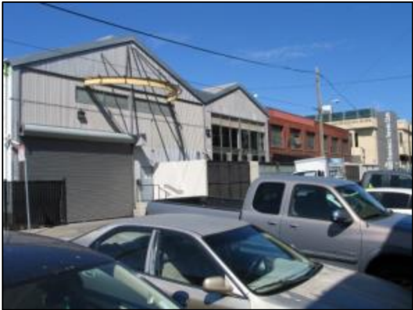
Photograph 133. Rear of ES-31, mid-block Bluxome Street, facing northeast.
