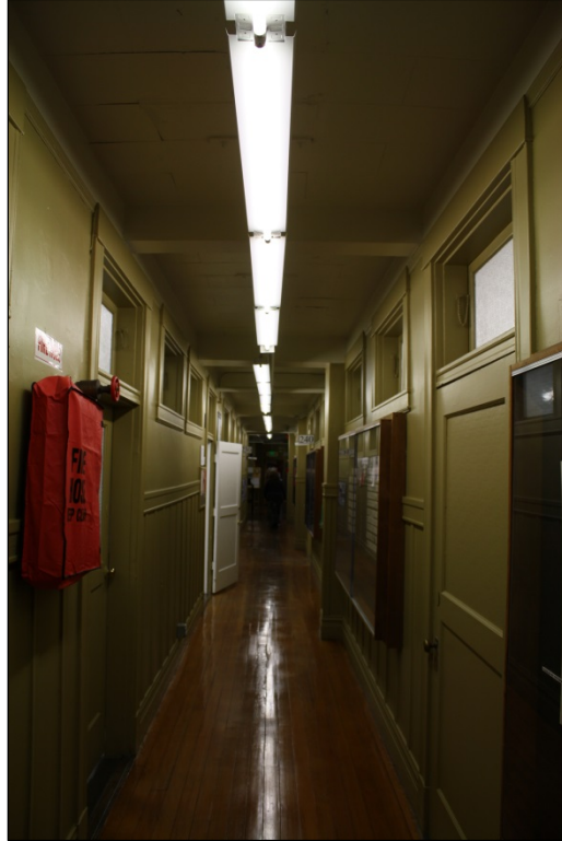
Figure 131. Example interior of subject property.
