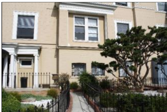
Photograph 49. South façade, 1916 Octavia Street
