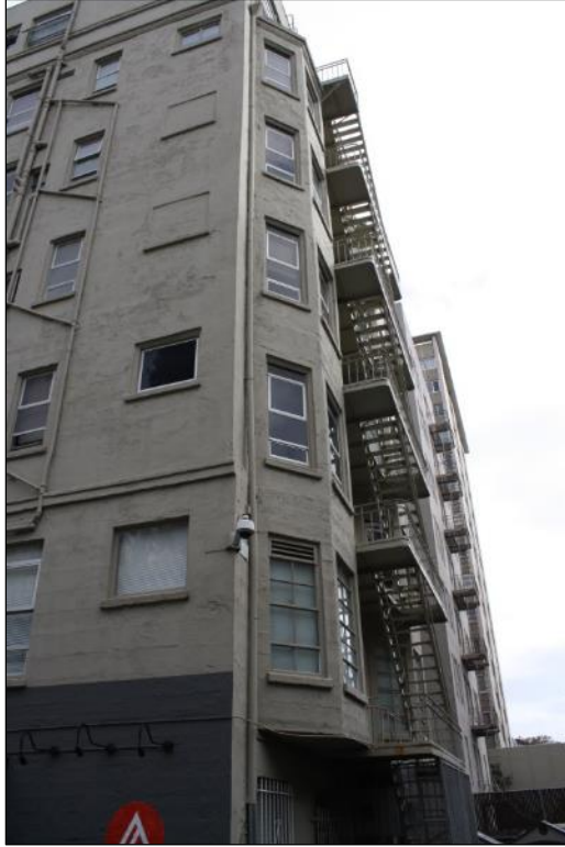
Figure 96. 1055 Pine Street, northeastern perspective, southwest corner. (Source: SWCA)
