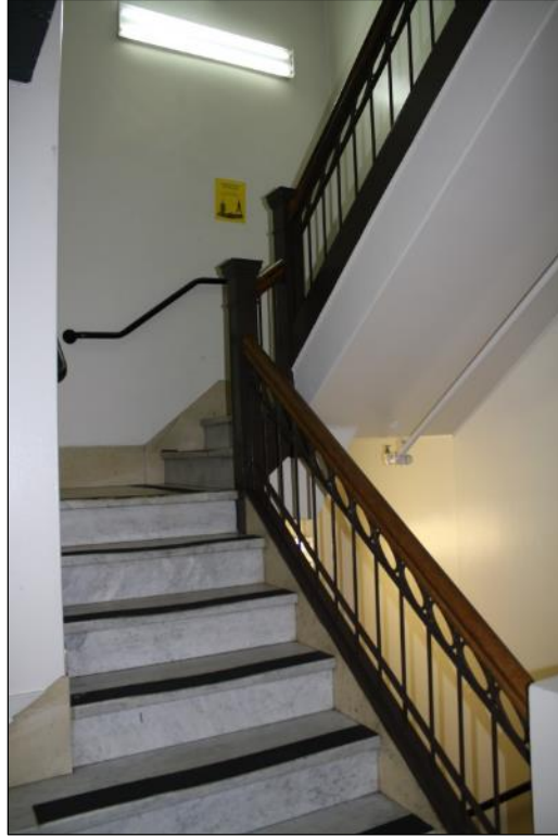
Figure 97. Interior view of the stair of subject property. (Source: SWCA)
