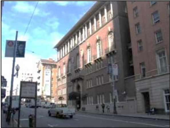
Photograph 100. Mid-block Sutter Street, facing northwest.
