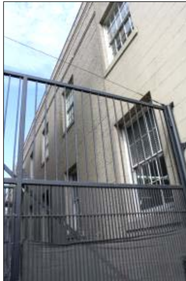
Photograph 141. 460 Townsend Street, detail of secondary elevation.
