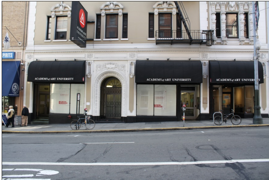
Figure 164. 625-629 Sutter Street, first story of the primary elevation.
