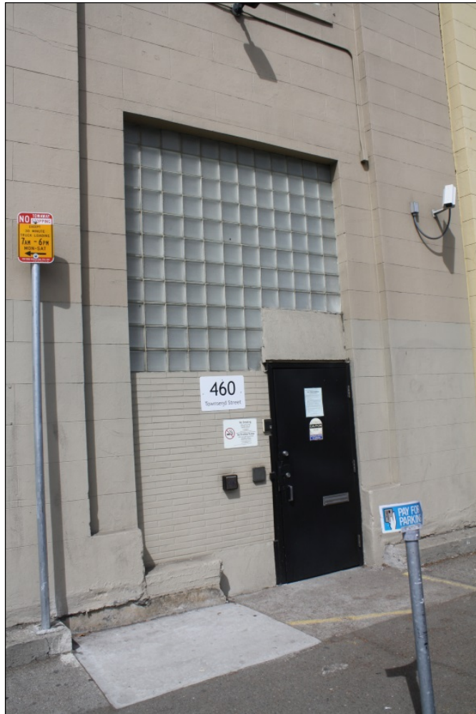
Figure 259. 460 Townsend Street, close up of the entry on the primary elevation.
