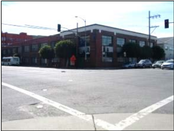
Photograph 132. 601 Brannan Street (ES-31).
