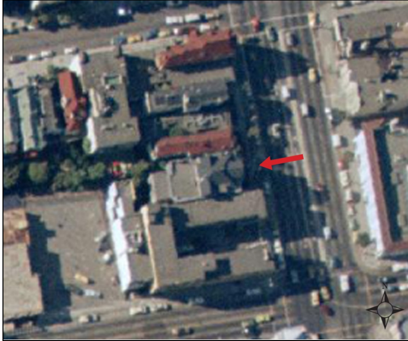
Figure 349. 1974 Aerial Photograph, 2209 Van Ness Avenue. (Source: Environmental Data Resources)
