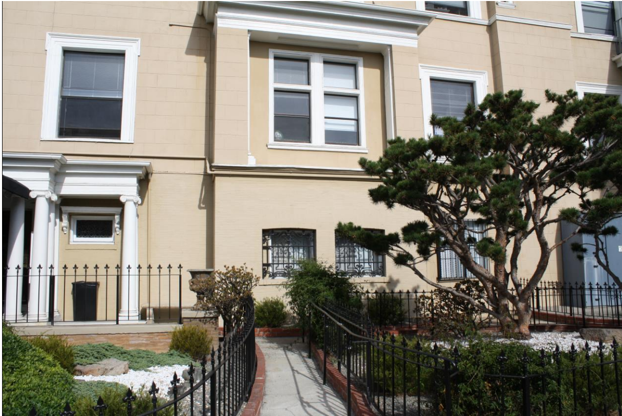
Figure 4. South façade, 1916 Octavia Street. Source: SWCA, 2015.
