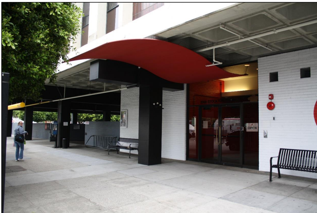
Figure 5. West façade, entrance detail, 2340 Stockton Street. Source: SWCA, 2015.
