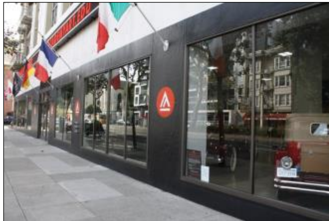
Photograph 42. 1849 Van Ness Avenue, detail of windows on ground level of primary elevation.
