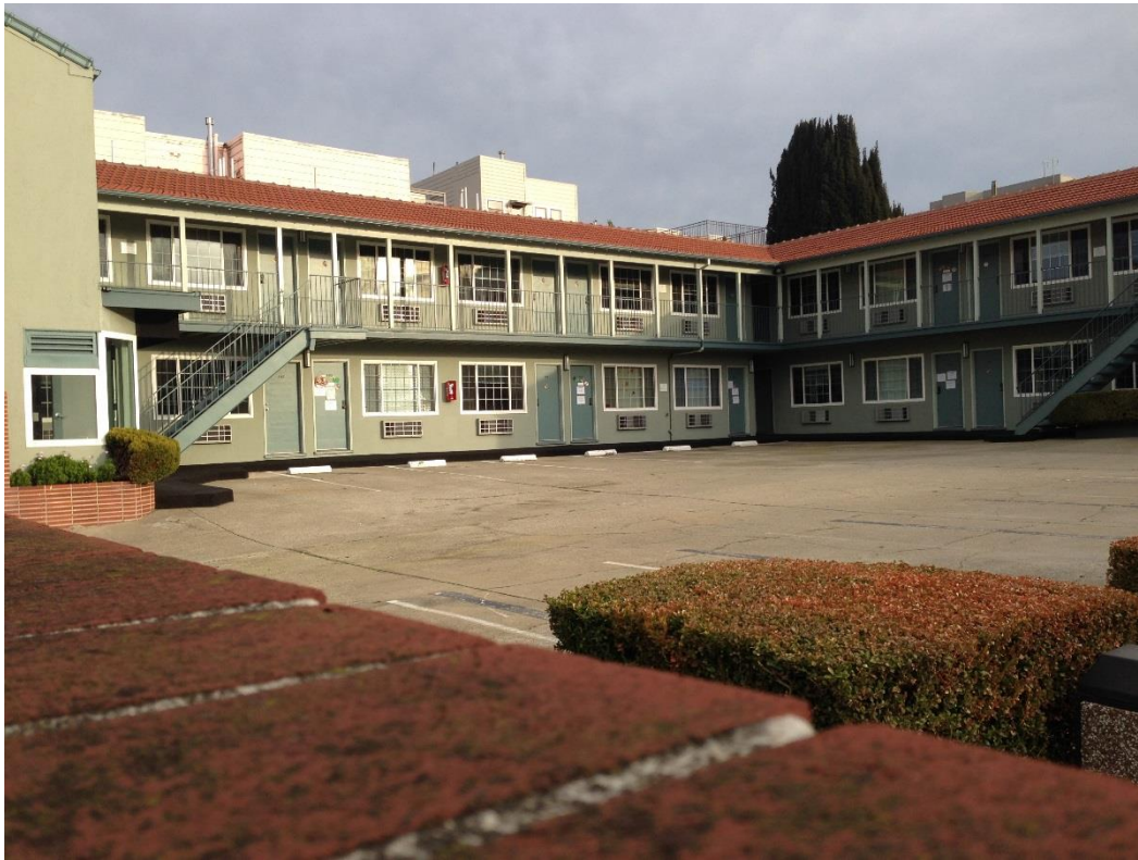
Figure 4. Eastern wing (1953), Star Motel, 1727 Lombard Street, 2015 (Source: SWCA).
