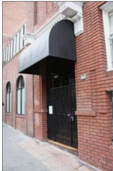
Photograph 60. 1153 Bush Street, detail of primary entrance.
