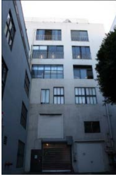
Photograph 131. 58–60 Federal Street, southwestern perspective of the northeastern elevation.
