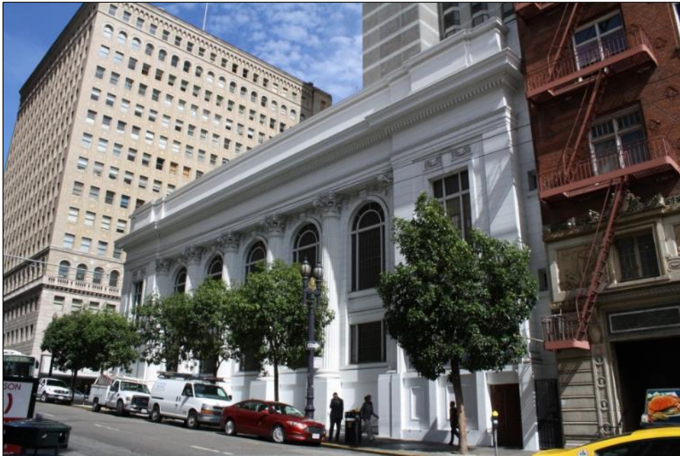
Figure 112. 491 Post Street, northeast perspective of the western elevation. (Source: SWCA)
