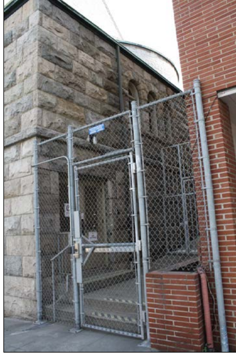
Figure 312. 2151 Van Ness Avenue, close up of the gate and entry door on the western elevation.
