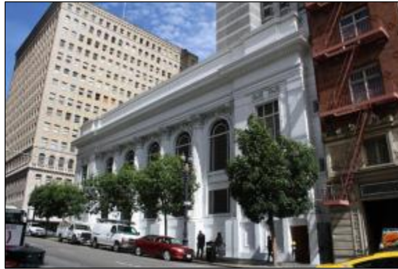
Photograph 109. 491 Post Street, Mason Street elevation.
