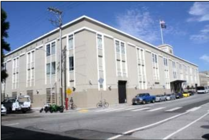
Photograph 142. 466 Townsend Street (ES-34).
