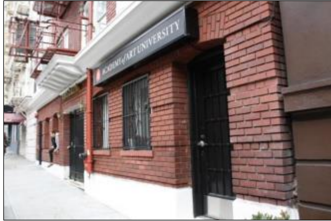
Photograph 67. 1080 Bush Street, detail of ground level.
