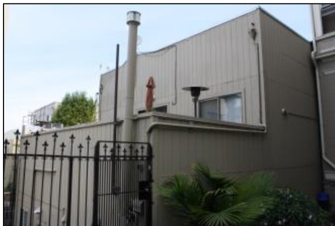
Photograph 26. 2211 Van Ness Avenue, northeastern perspective of the upper stories of the west elevation
