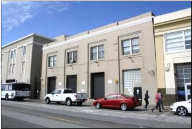
Photograph 136. 460 Townsend Street (ES-33).
