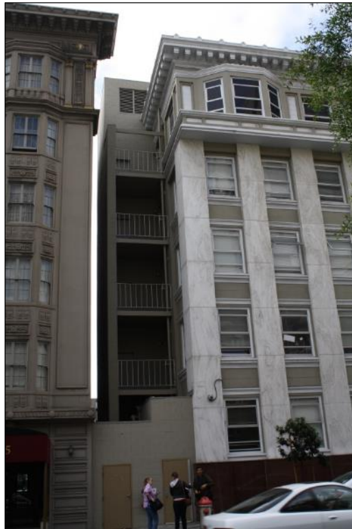
Figure 93. 1055 Pine Street, detail, fire stair case addition on the primary elevation. (Source: SWCA)
