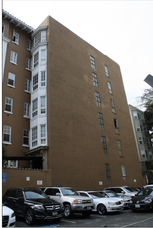
Figure 192. 680 Sutter Street, northwestern perspective of the northern portion of the eastern elevation.
