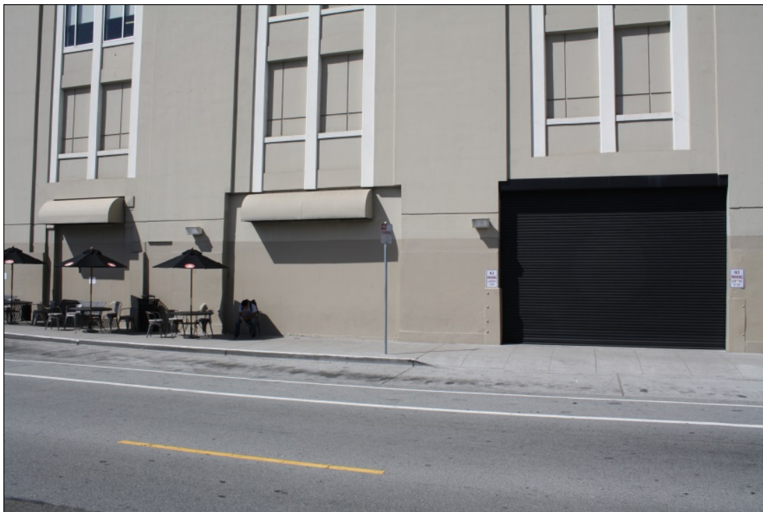
Figure 273. 466 Townsend Street, close up of the roll-doors and in fill on the northern half of the primary elevation.
