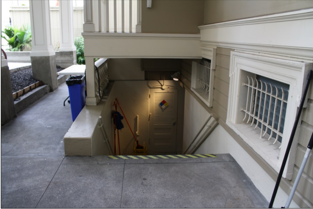
Figure 338. 2209 Van Ness Avenue, close up of the basement entry and windows on the west elevation.
