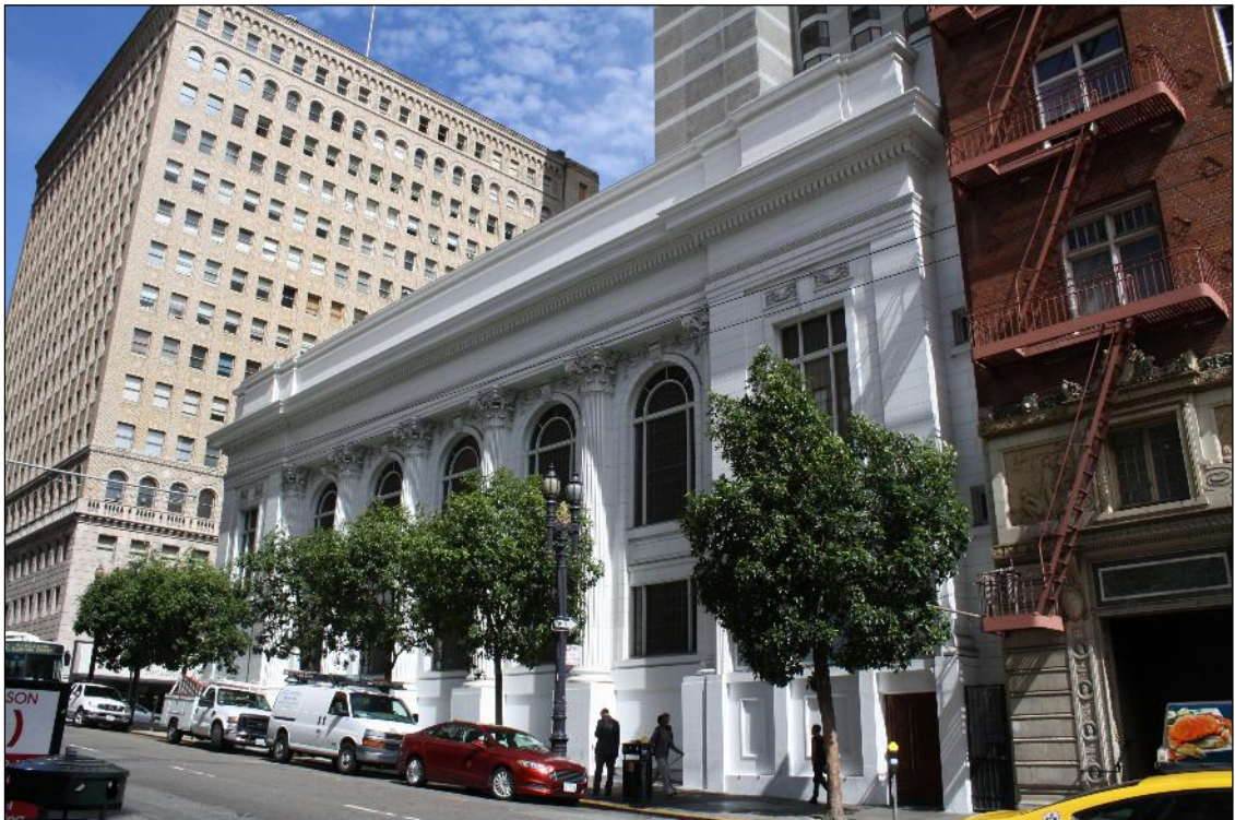
Figure 108. 491 Post Street, Mason Street elevation, southwest perspective. (Source: SWCA)
