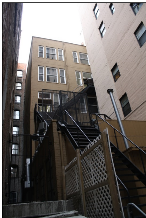
Figure 166. 625-629 Sutter Street, western perspective of the south and rear eastern elevations.
