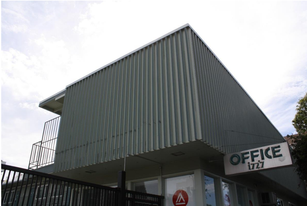
Figure 6. Office wing, Star Motel, 1727 Lombard Street, 2015 (Source: SWCA).
