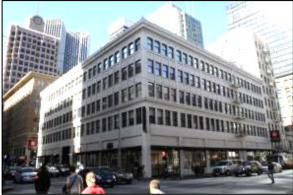
Photograph 111. 77 New Montgomery Street (ES-27).
