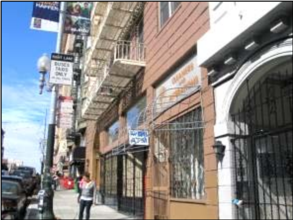
Photograph 71. Mid-block Sutter Street, facing northwest.
