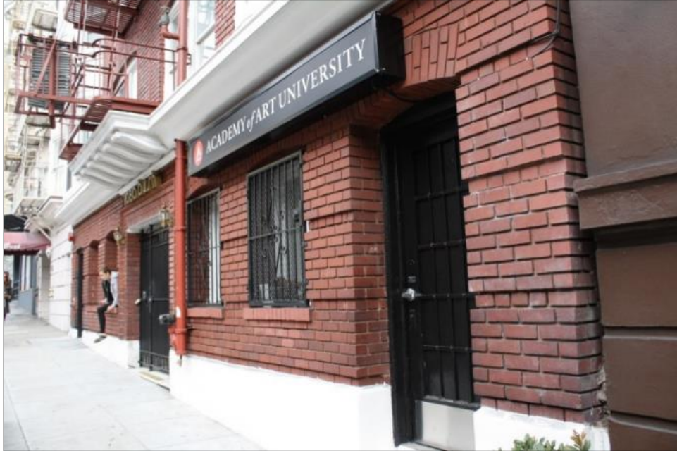
Figure 15. 1080 Bush Street, detail, first story of the primary elevation. (Source: SWCA)
