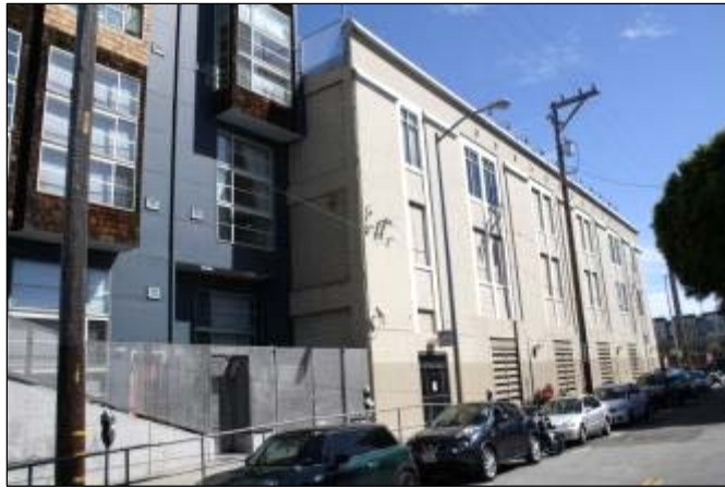
Photograph 147. 466 Townsend Street, secondary elevation.
