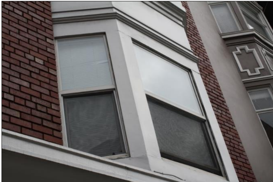
Figure 16. 1080 Bush Street, detail, projecting bay windows of the primary elevation. (Source: SWCA)
