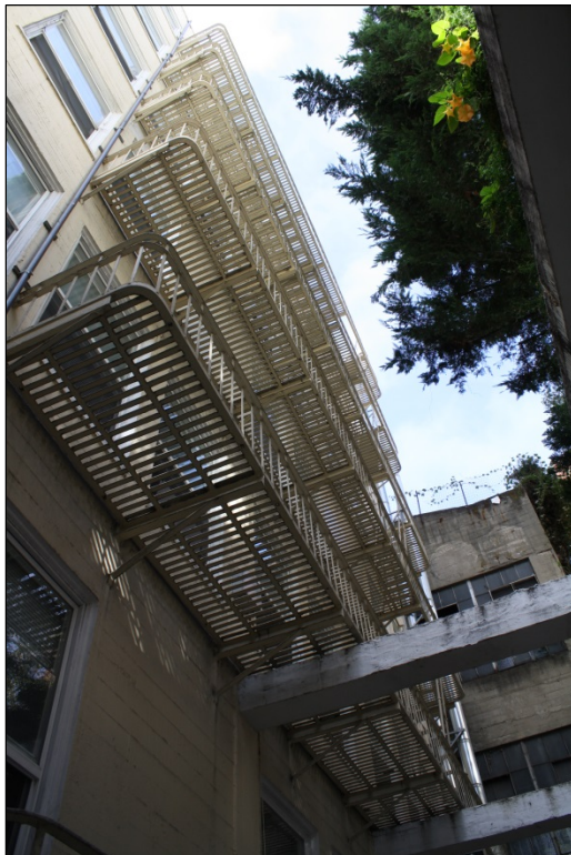
Figure 232. 860 Sutter Street, southwestern perspective of the north elevation.
