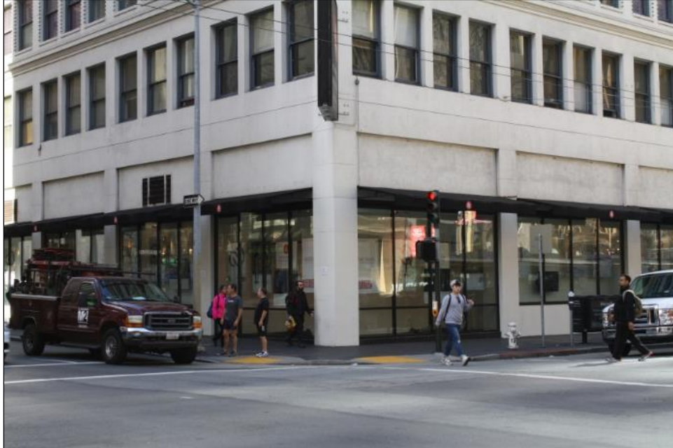
Figure 59. 77-79 New Montgomery Street, detail, storefronts on the first story. (Source: SWCA)
