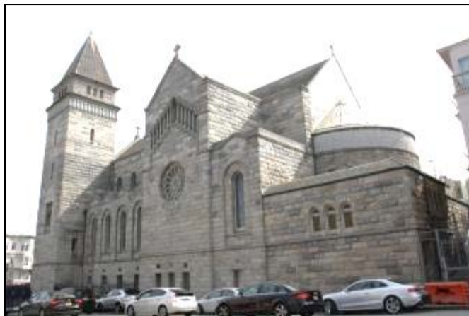
Photograph 35. 2151 Van Ness Avenue, southeastern perspective of the north and west elevations
