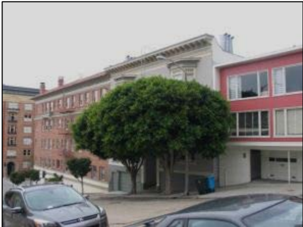
Photograph 46. Mid-block Octavia Street, facing southwest.
