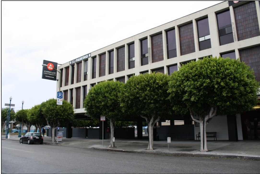
Figure 4. West façade, 2340 Stockton Street. Source: SWCA, 2015.
