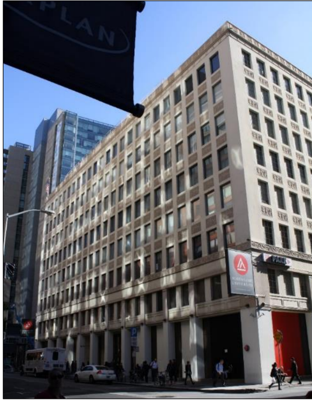
Figure 85. 2015 photograph of 180 New Montgomery Street. (Source: SWCA)
