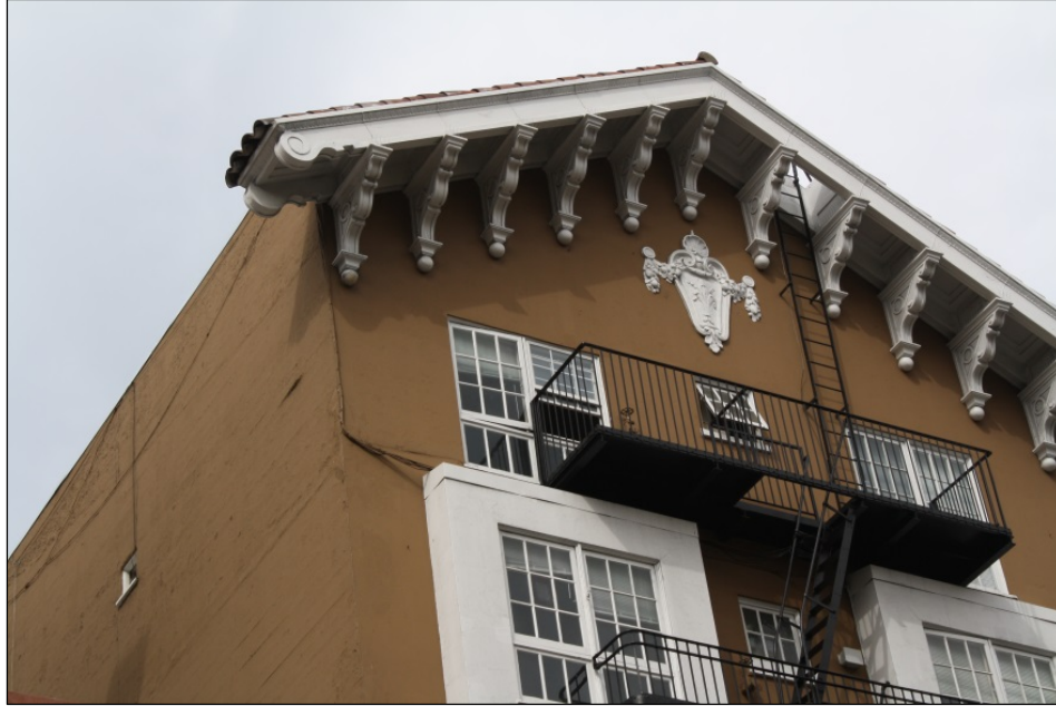
Figure 194. 680 Sutter Street, northeastern perspective of the west and primary (south) elevations.
