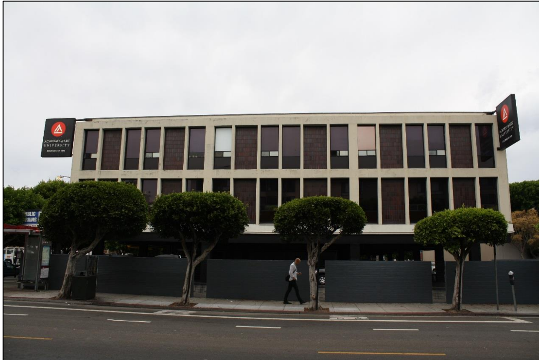
Figure 7. South façade, 2340 Stockton Street. Source: SWCA, 2015.
