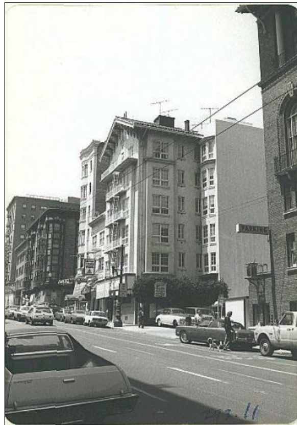
Figure 199. 1976 photo of 680 Sutter Street. (Source: San Francisco Heritage)
