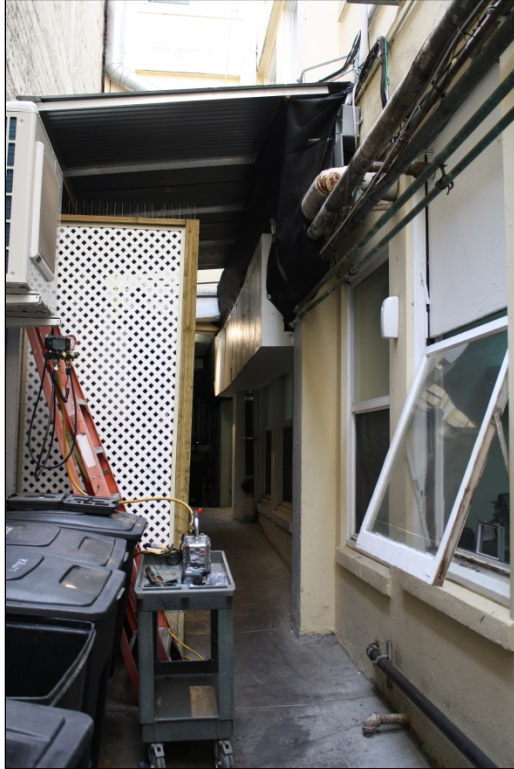
Figure 231. 860 Sutter Street, southern perspective of the first floor on the eastern elevation.
