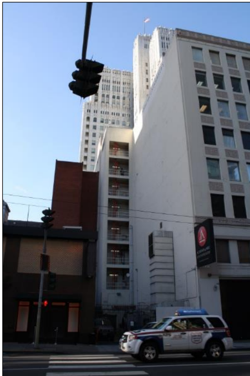
Figure 79. 180 New Montgomery Street, northwestern perspective of the southwest elevation. (Source: SWCA)
