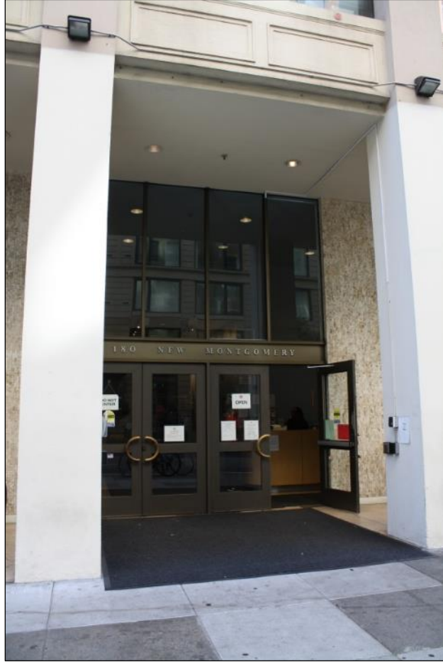
Figure 75. 180 New Montgomery Street, detail, main entry on the primary elevation. (Source: SWCA)
