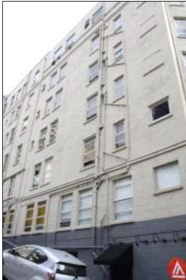
Photograph 95. 1055 Pine Street, northeast perspective, west elevation.
