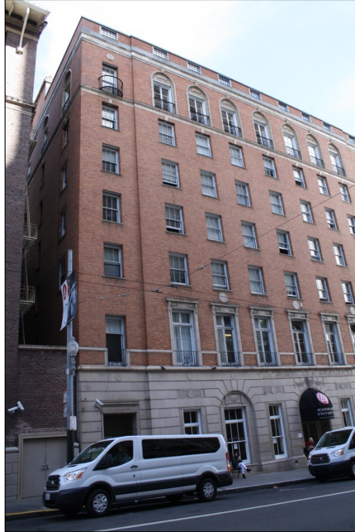
Figure 152. 620 Sutter Street, northern perspective of the south and west elevations.
