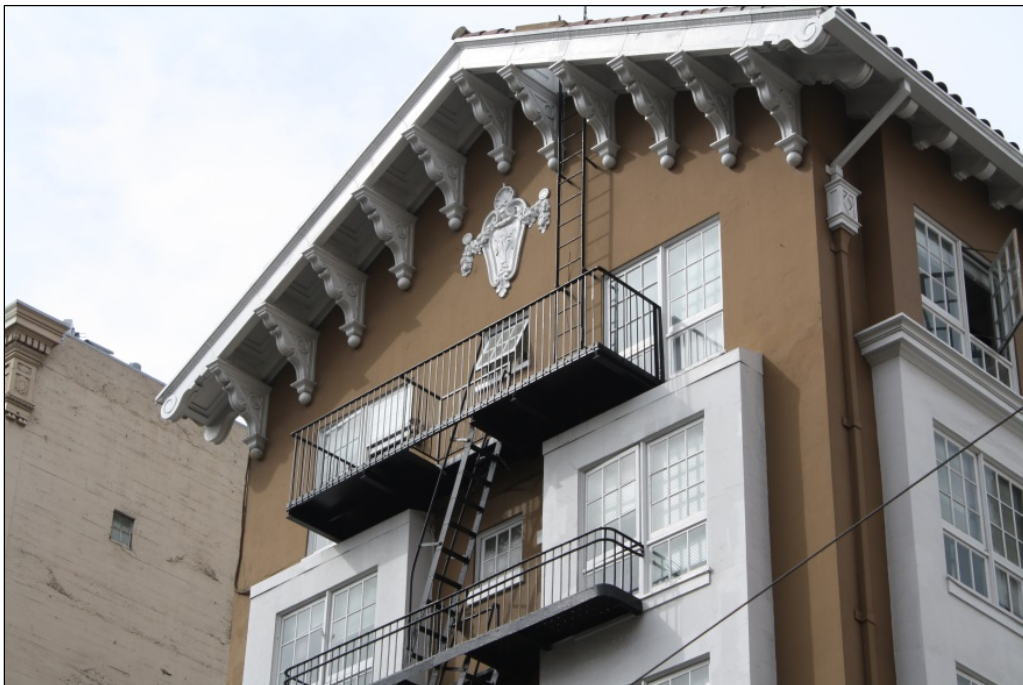
Figure 188. 680 Sutter Street, close up of the decorative brackets and rafter ends on the primary elevation.
