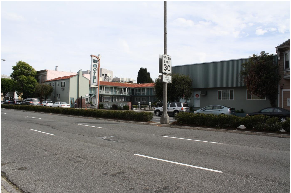
Figure 3. Contextual view of Star Motel, 1727 Lombard Street, 2015 (Source: SWCA).
