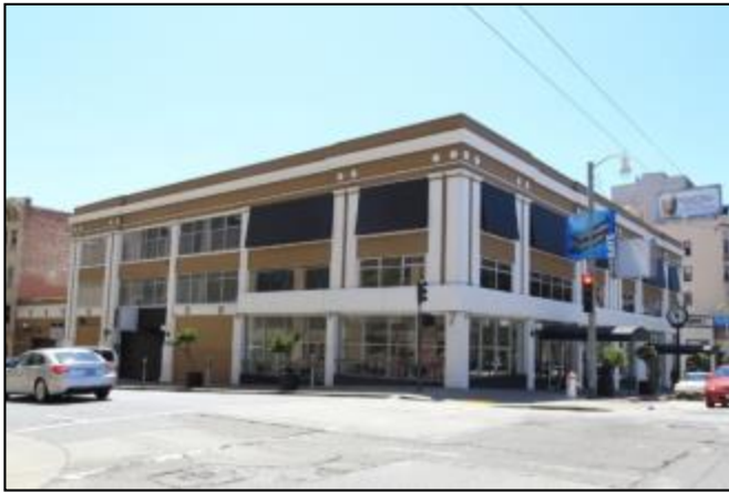
Photograph 51. 950 Van Ness Avenue (ES-10).
