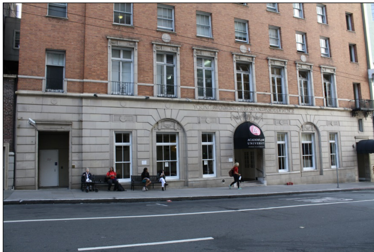
Figure 149. 620 Sutter Street, first and second story of the primary elevation.
