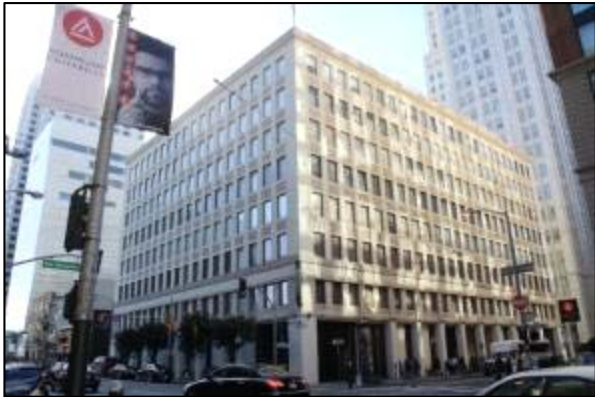
Photograph 118. 180 New Montgomery Street (ES-28).
