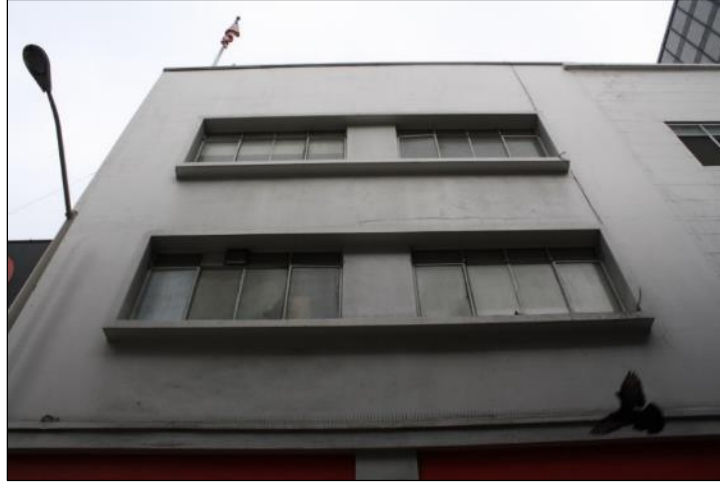
Figure 3. 410 Bush Street, close up of ribbon casement windows on the east elevation. (Source: SWCA)
