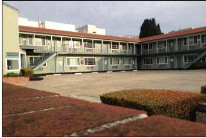
Photograph 19. Eastern wing (1953), Star Motel, 1727 Lombard Street
